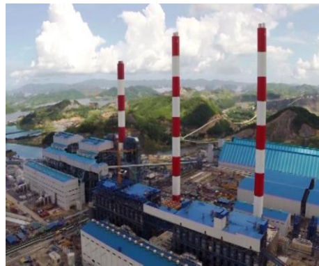
Mong Duong 2 TCP plant
