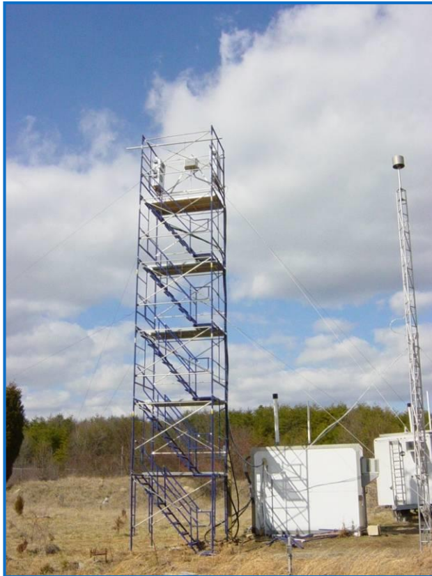
Beltville, Maryland mercury site
