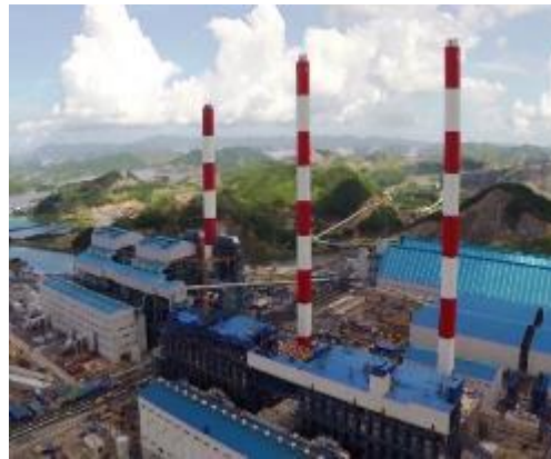
Mong Duong 2 TCP plant
