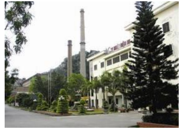
Ninh Binh TCP plant
