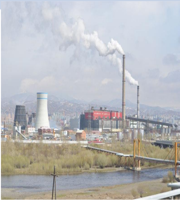
TERMO POWER PLANTS(TPP) HEAT ONLY BOULERS (HOBs)
