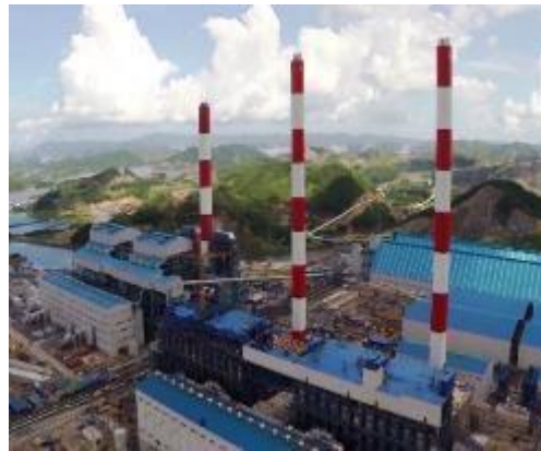
Mong Duong 2 TCP plant
